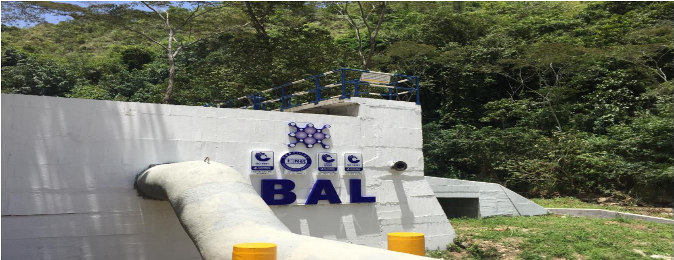
Bocatoma IBAL S.A. E.S.P.
